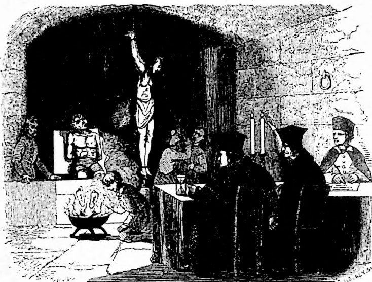
TORTURES OF THE PULLEY AND THE FIRE.
