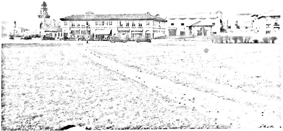
74. Spanish Revival came to Kansas City in 1923, with the construction of Country Club Plaza. Courtesy, Missouri Valley Special Collections, Kansas City Public Library, Kansas City, Missouri.
